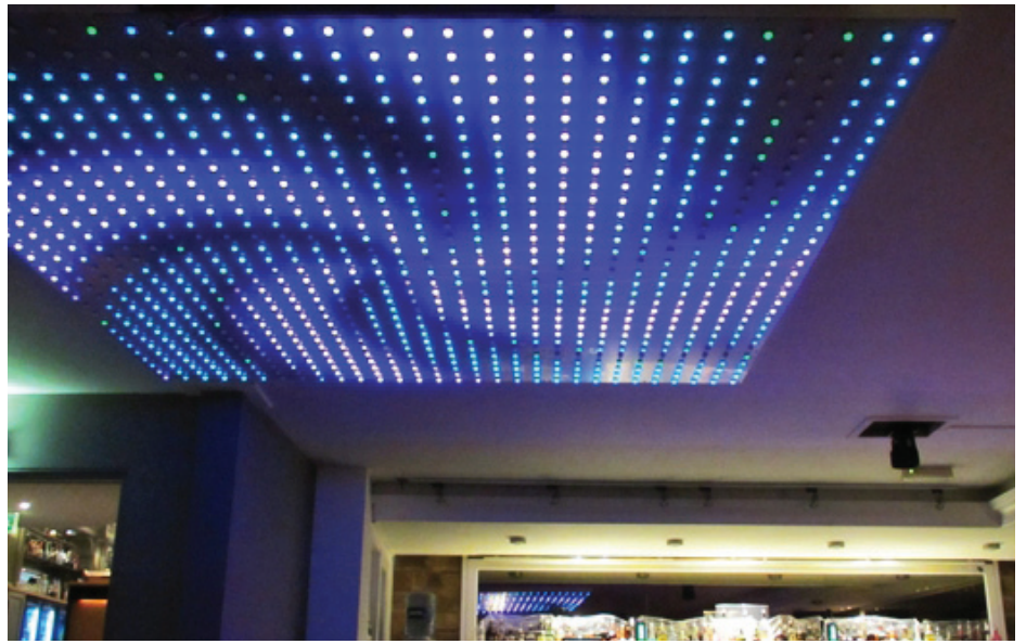
Dome20 Ceiling Installation
